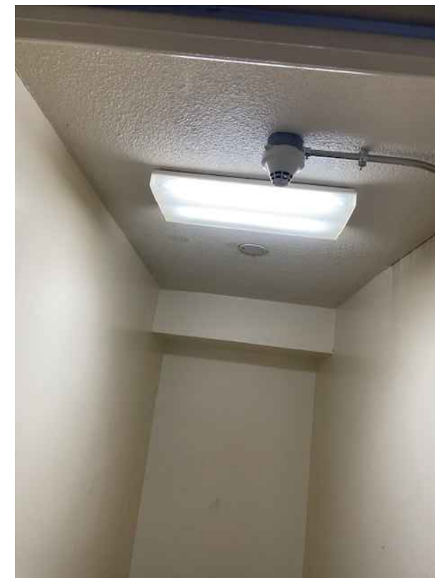
Picture 1: Gypsum ceiling with textured ACM identified.
